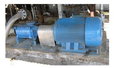
The plant asked Azima DLI to take baseline vibration readings from the spare pump and then perform periodic surveys to ensure proper operation. This was the site's only spare and if it also failed, it would cripple plant production by 50 percent for approximately 48 hours.
